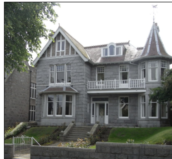
Building may exhibit a variety of window sizes and glazing patterns. This can provide important evidence of the history of the building and contribute to its character and interest
