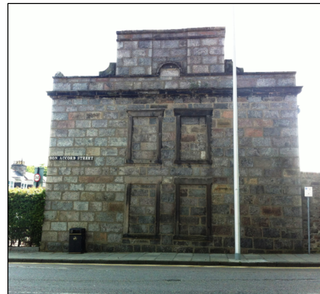
Example of blocked up windows in Ferryhill
